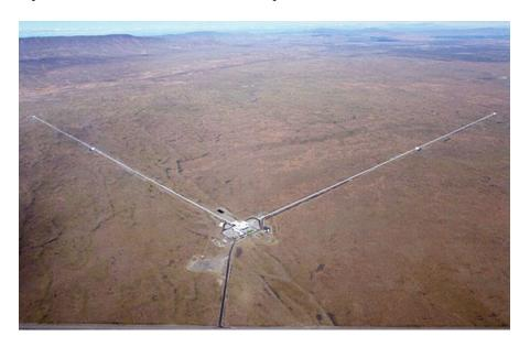
LIGO's antennas are L-shaped, with perpendicular arms 2.5 miles long. Inside each arm, cocooned in layers of steel and concrete, runs the world's largest bottle of nothing, a vacuum chamber a couple of feet wide containing 2.5 million gallons of empty space. At the end of each arm are mirrors hanging by glass threads, isolated from the bumps and shrieks of the environment better than any Rolls-Royce ever conceived.
